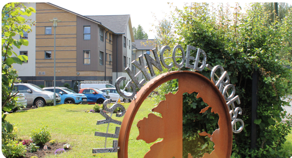
Above: The front entrance to Llys Glyncoed Care Home, with the new, slate look Metrotile Woodshake roof in the background.
